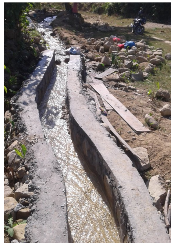
Irrigation Canal constructed in Bhulke community, Dang
